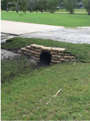
Figure 9. Driveway Culvert Installation
