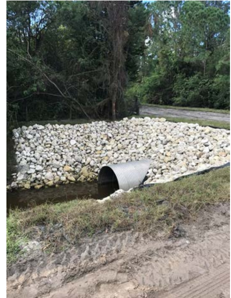
Figure 10. Canal 6 Culvert Installation
